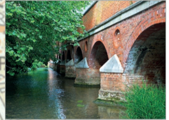
Arches under the town bridge
